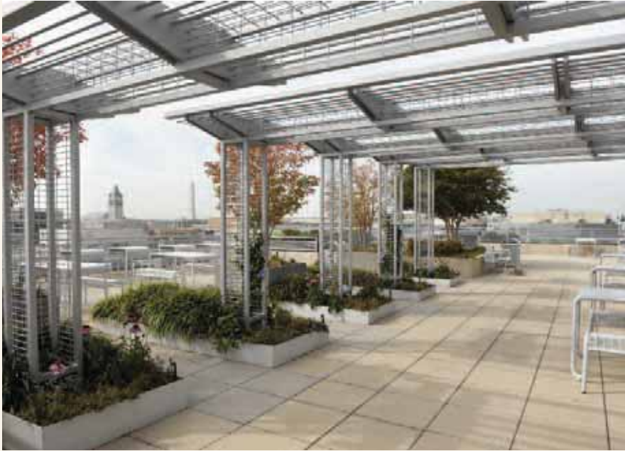
PHI's Edison Place headquarters features a 'green roof' that filters pollutants before runoff joins Washington's water system.
