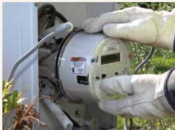
Installing a smart meter on a customer's home.
